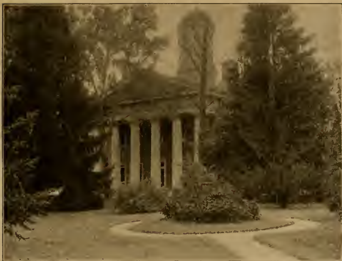
COURT HOUSE AT TOWSON.
